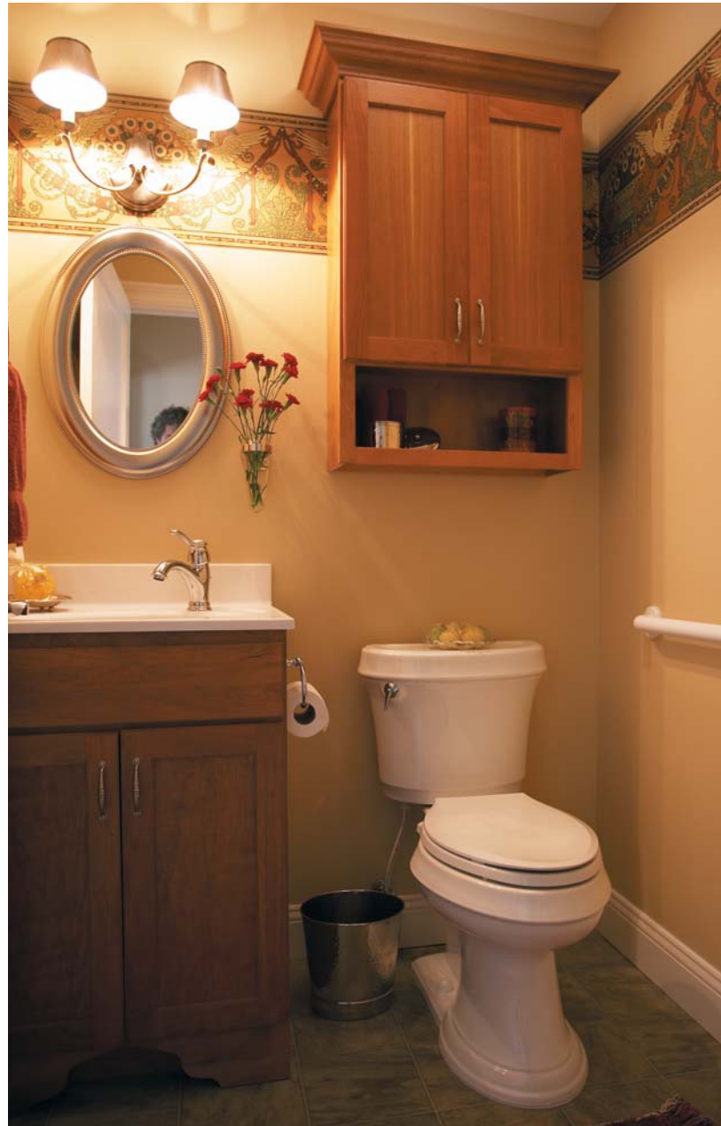
The home's powder room includes accessible features such as a 36-inch height vanity to minimize bending and a three-foot wide doorway.
